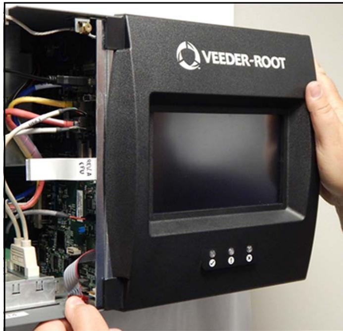
Figure 21. Install The New TLS-450PLUS Display Door
